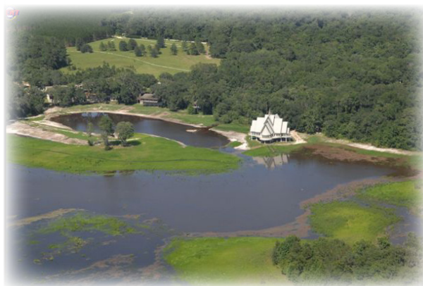
Aerial view of Camp Weed
