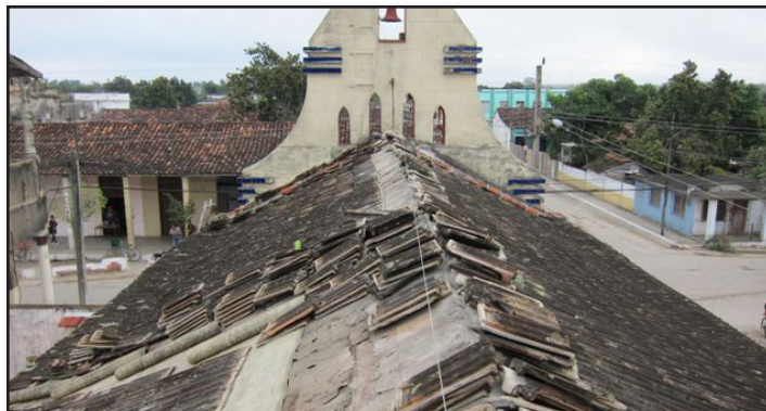
The photo above shows the degraded condition of the roofing material as it was removed from the church. The above right photo shows the new and improved, water-tight roof.
