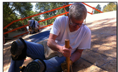
Cliff Taylor (foreground) works on the roof.
