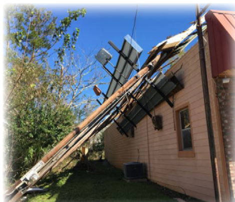
A billboard in its entirety was deposited onto this home.
