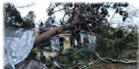
Two homes were crushed by one tree.
